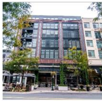
Mixed Residential over Commercial
